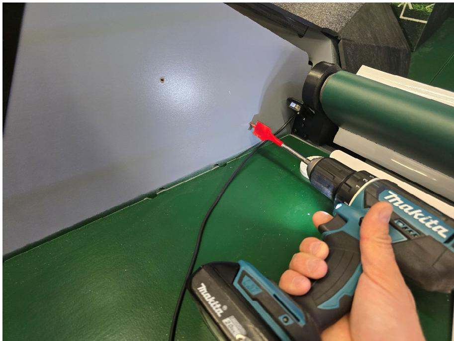
**Step 13:** Insert the sensor harness into the left chamber (where you just drilled the hole). Connect the extension harness to the sensor.
